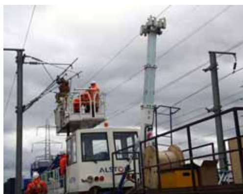
Telescopic mast, sq. 300 mm, h= 3,00-5,00 m
