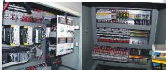
MAIN AND SECOND ELECTRIC BOARDS
